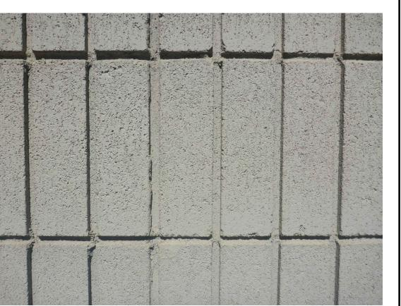
8"x8"x16" CONCRETE MASONRY BLOCK, COLOR AND PATTERN AS SHOWN TO MATCH
